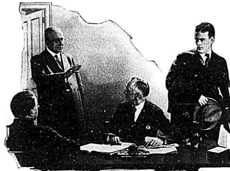
Scene: Superintendent's Office. Characters, left to right: Plant Engineer; President; Superintendent; JOHNSON Sales Engineer.
