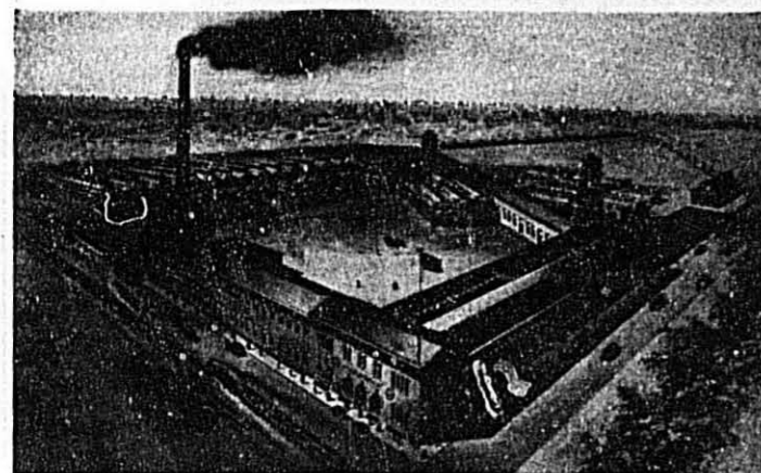
Plant at Summerdale, Philadelphia
